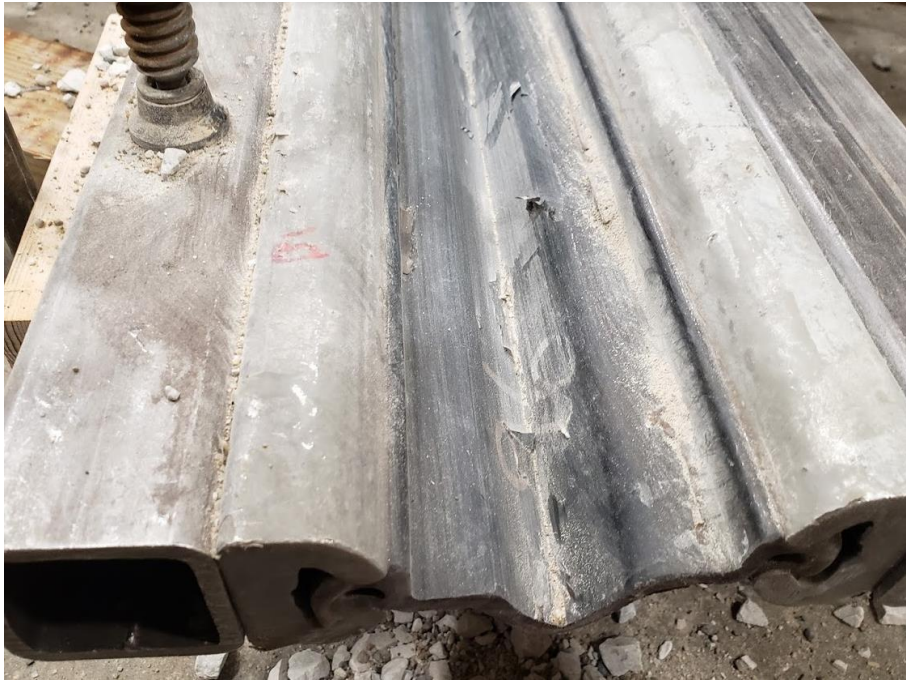
Figure 28: No Apparent Damage Following Testing
